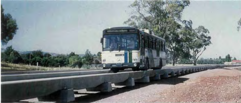
The Mercedes-Benz O-Way System shows the proven rail-guided buses. Part of the 8-mile long O-Way track in Adelaide, Australia.
