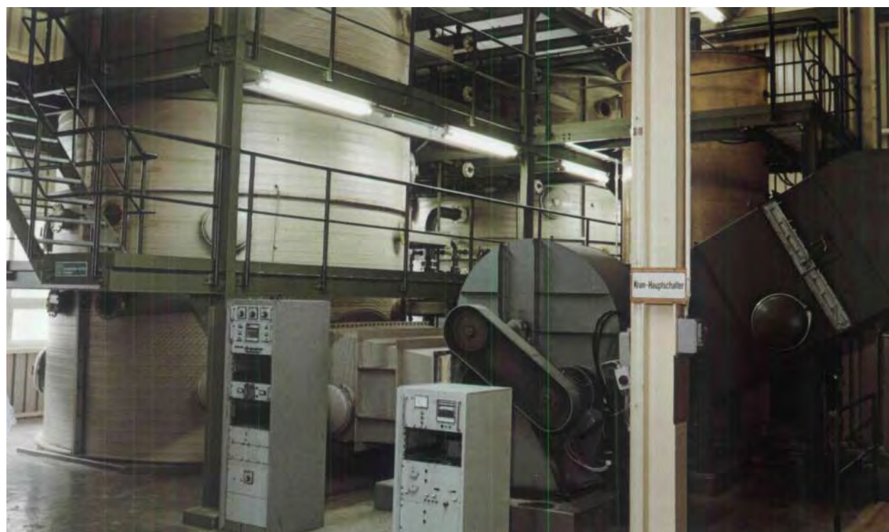
Biological air cleaning systems in Mettingen. Every hour approximately 4.2 million cubic feet of foundry air is cleaned. Even the water required by the system is cleaned with the aid of micro organisms and is recirculated.
